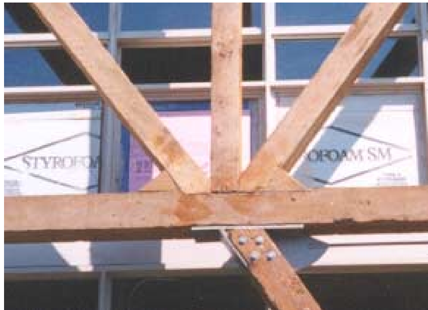
Extruded polystyrene insulation at the Materials Testing Lab
