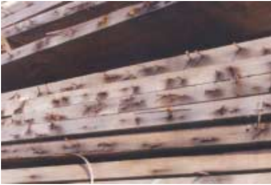
Joists prior to denailing
