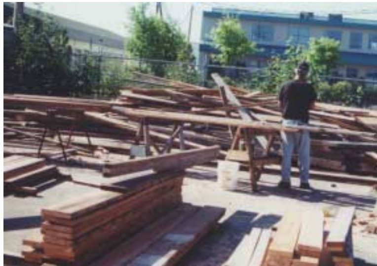
Denailing and sorting salvaged wood. Bent Nail salvaged materials yard, Abbotsford
