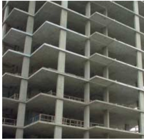
Non-combustible buildings in the Lower Mainland are typically framed with concrete and tend to have fewer salvageable materials.
