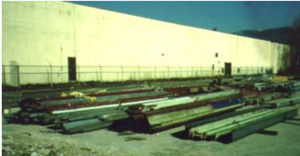
Salvaged wide- flange beams
