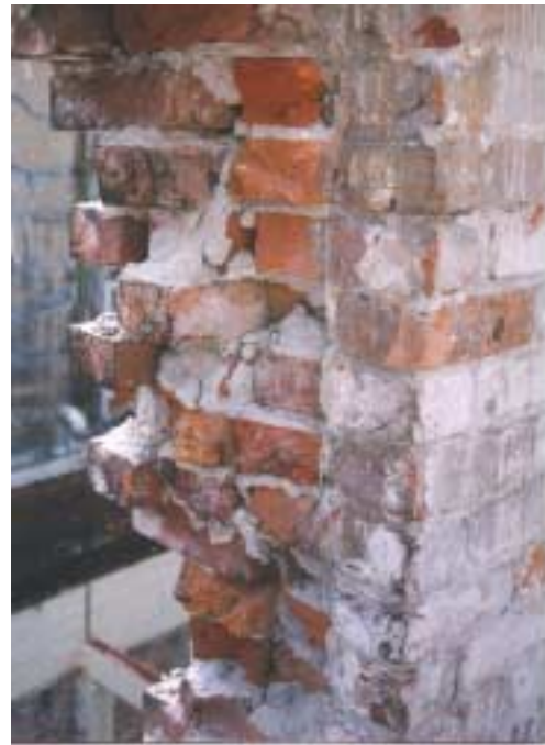
Salmon bricks used in the interior of a warehouse wall
