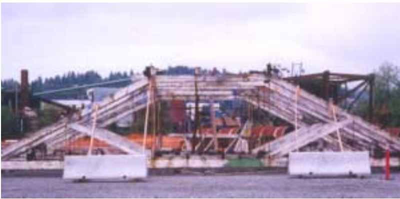
Trusses after removal from the Flavelle Cedar Mill
